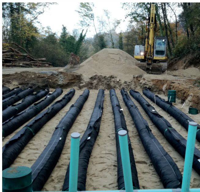
The rows of Advanced Enviro))Septic pipes
