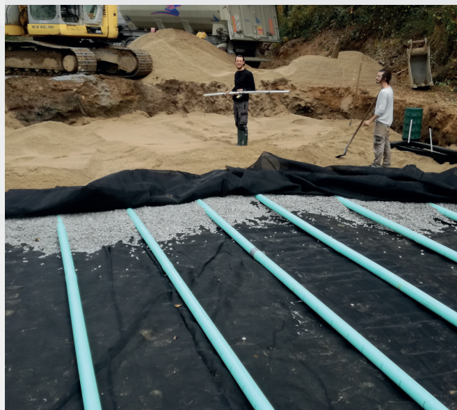
Laying the collection pipes and geogrid
