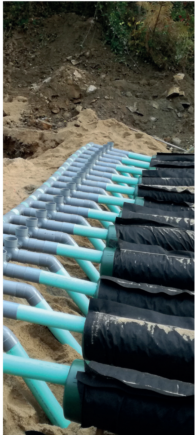
Installing the Low Pressure Repartition System Headers
