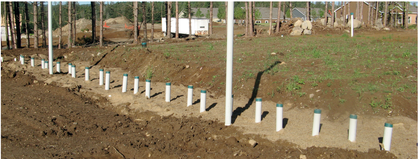
Ventilation and Low Pressure Repartition System headers
