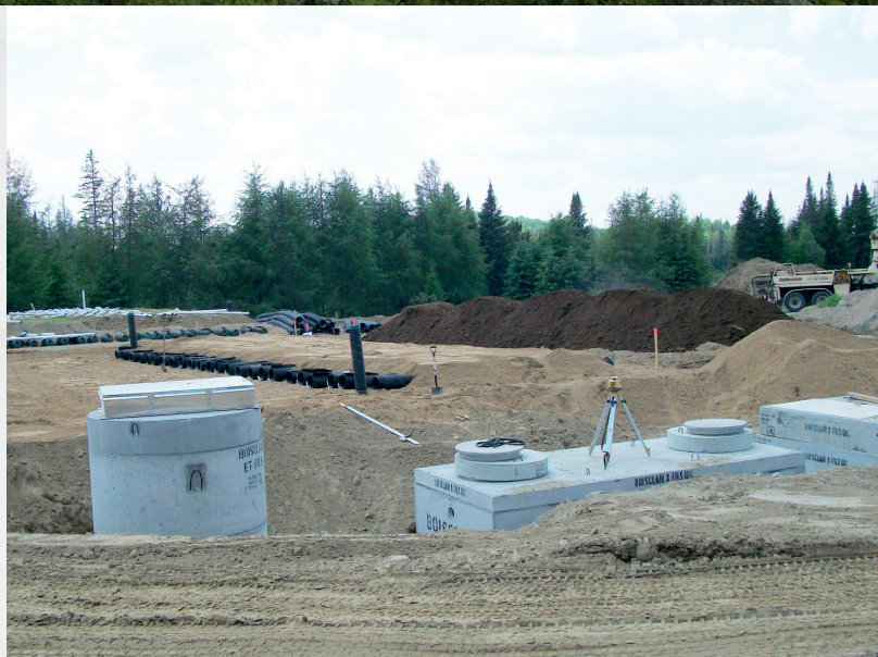
Septic tank and pumping station
