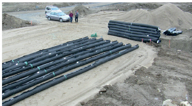
Rows of Advanced Enviro))Septic pipes
