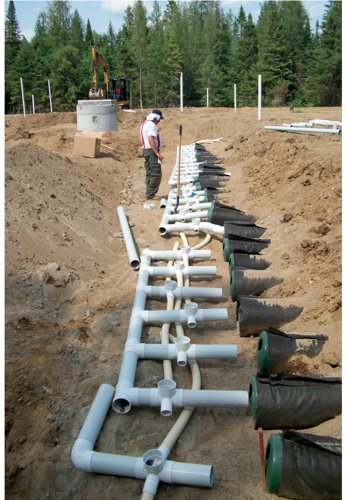
Attaching the Low Pressure Repartition System headers
