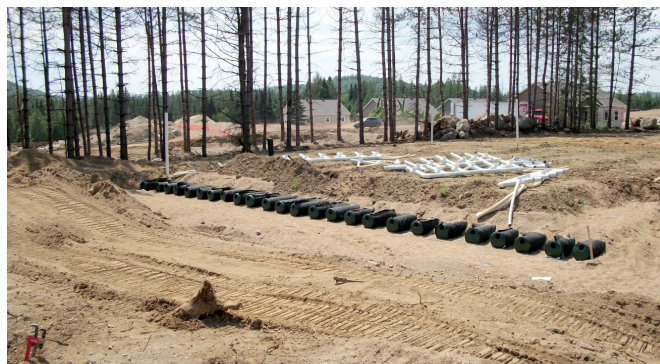
Covering the Advanced Enviro))Septic pipes with filter sand
