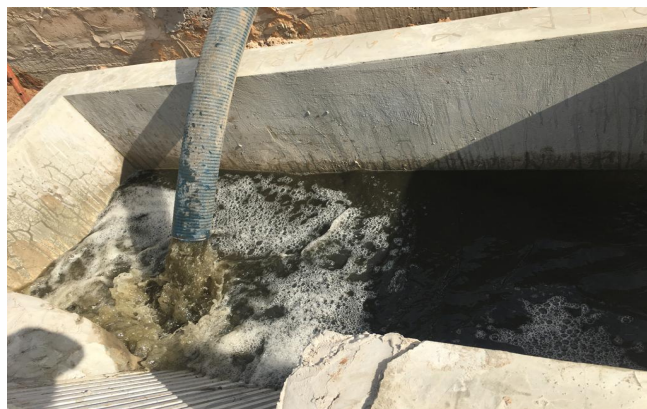
Wastewater discharged by a dump truck into a receptacle equipped with a bar screen built upstream of the System O))
