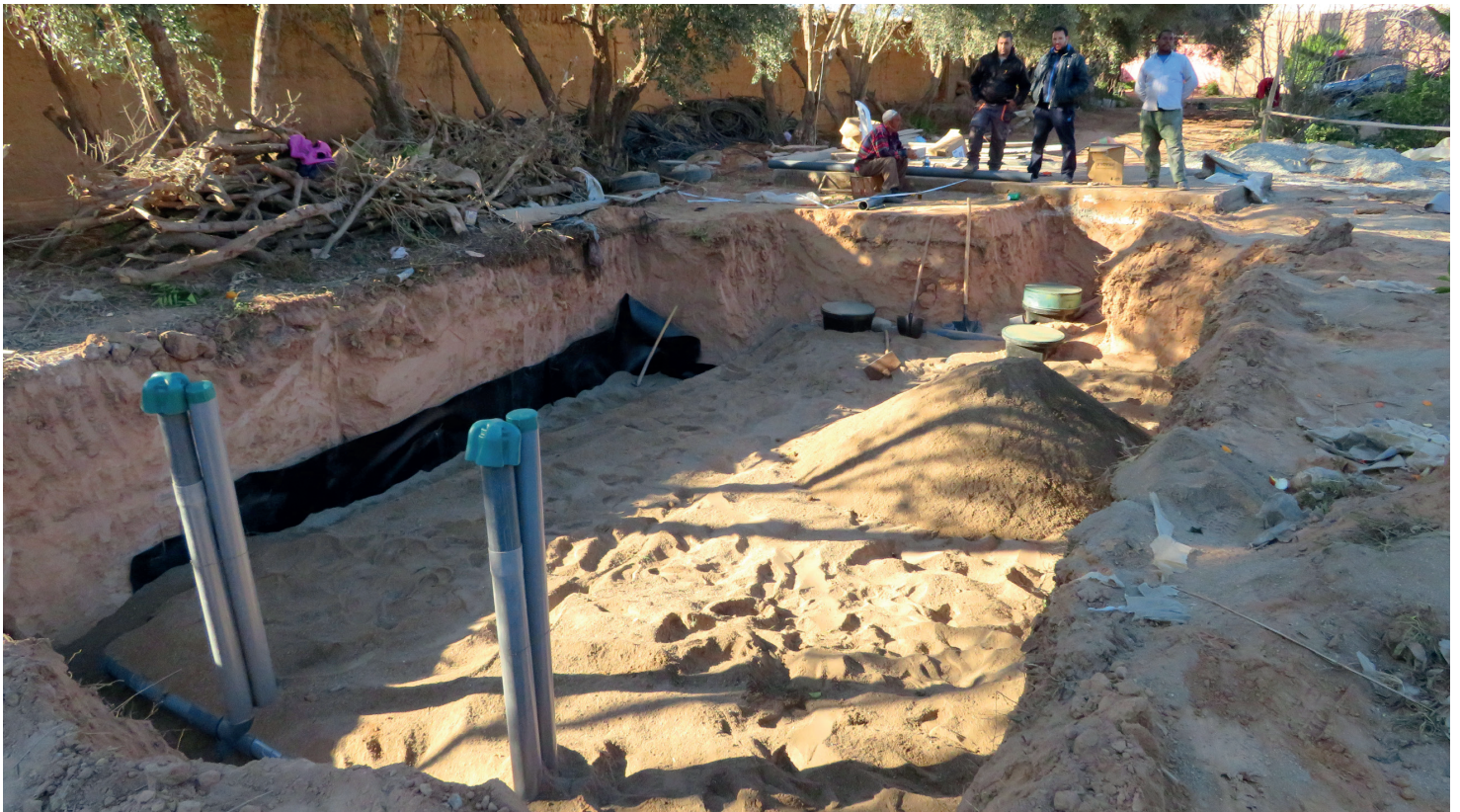
Covering the AES pipes and watertight membrane with filter sand and backfill
