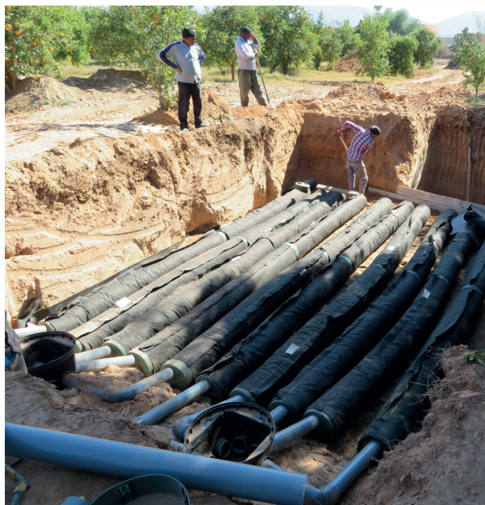
The connected AES pipes
