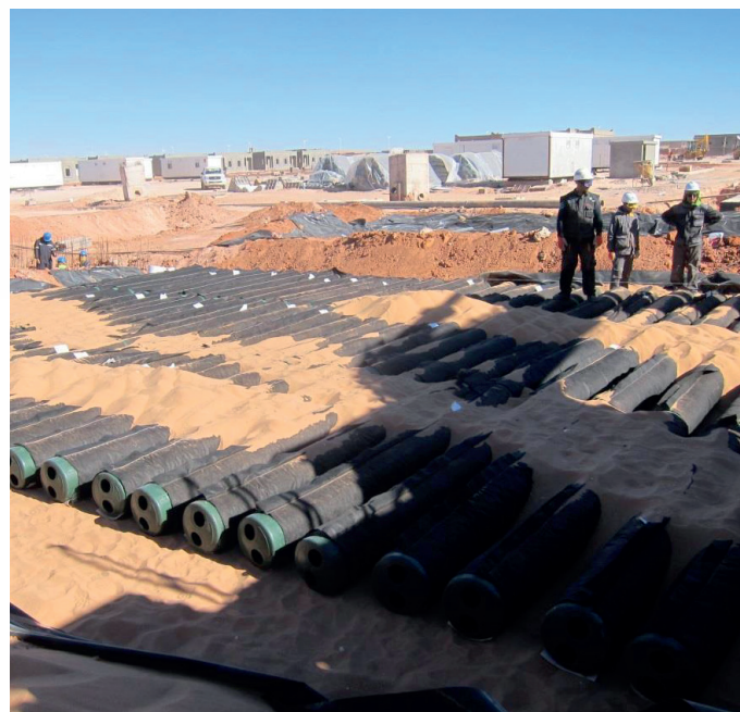
Covering the pipes with filter sand
