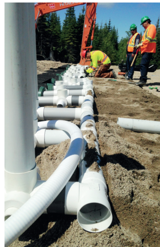
A low pressure distribution system
