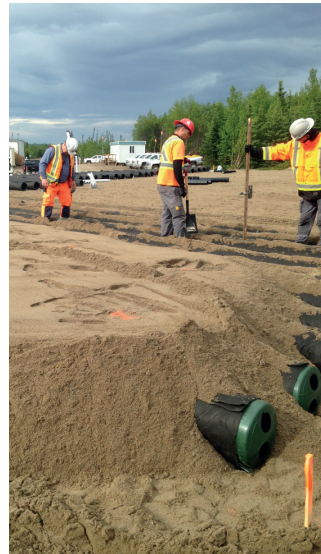
Covering the Advanced Enviro))Septic pipes with system sand
