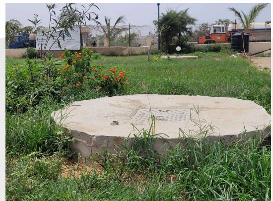
3000L tanks, one serving as a septic tank and the other as a storage tank for treated water
