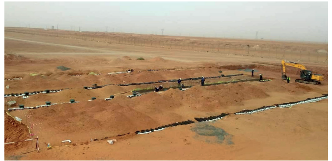
Pipes mostly covered by filter sand
