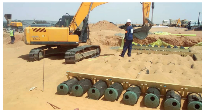
Holding the pipes in place while placing filter sand
