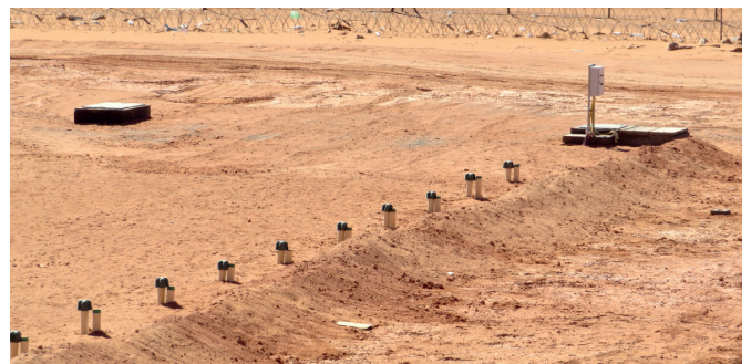
Control panel, piezometers and vents
