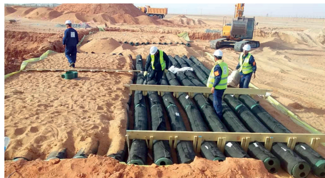
Holding the AES pipes in place while placing filter sand
