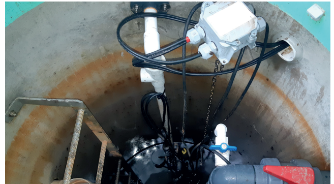
Pumping station that supplies water to the low-pressure headers
