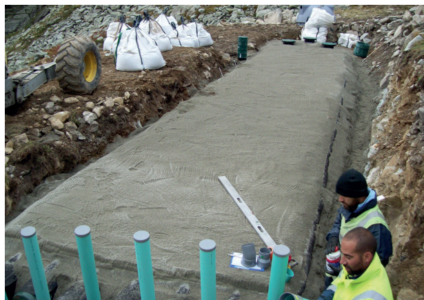
Covering the System O)) with filter sand
