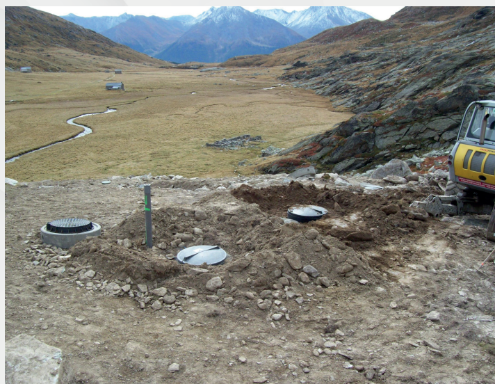
Grease trap and septic tank
