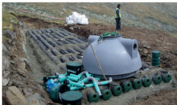
Placement of the septic system components
