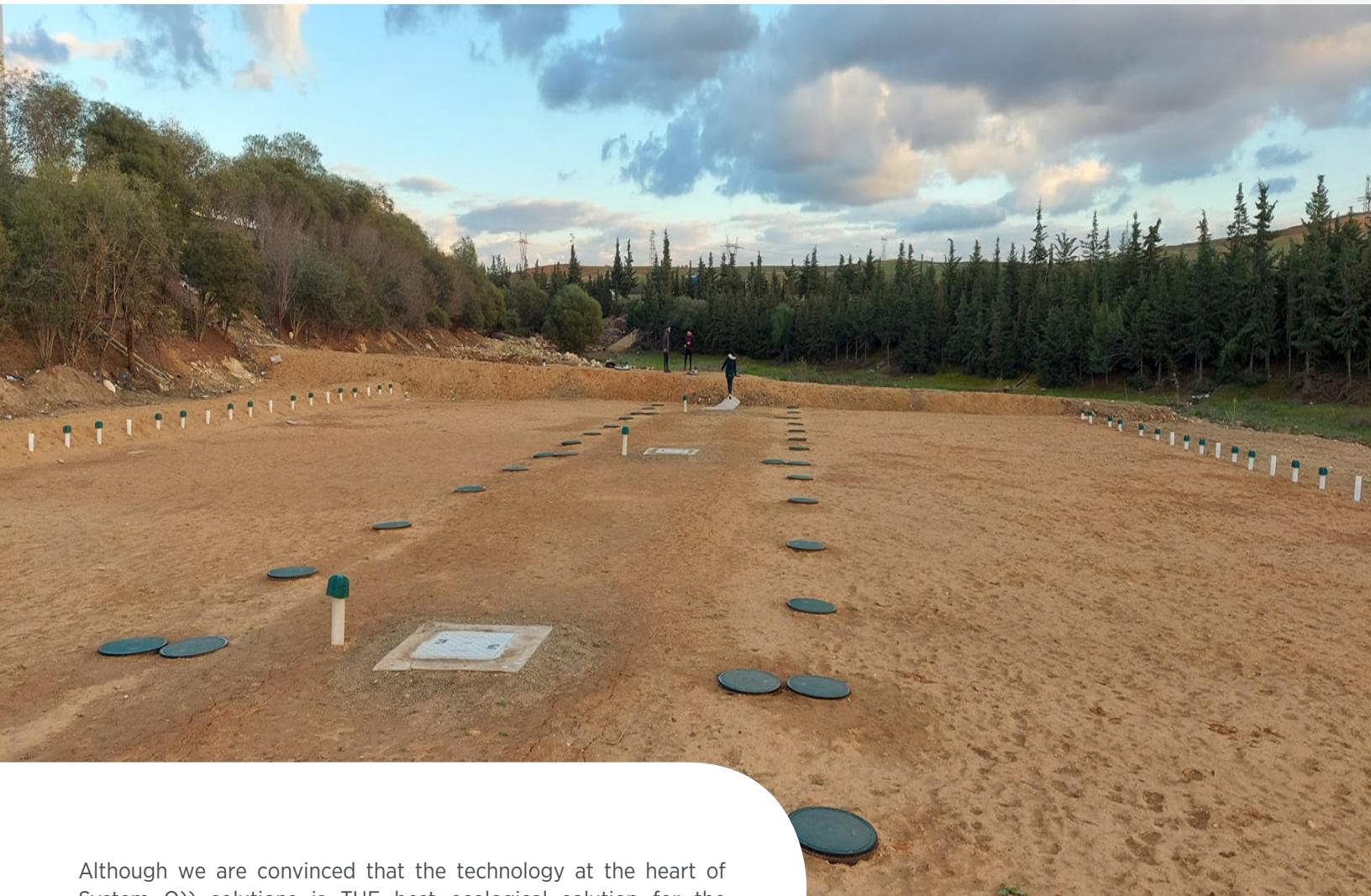
Although we are convinced that the technology at the heart of System O)) solutions is THE best ecological solution for the treatment of domestic wastewater, in some cases it can be difficult to take advantage of sufficient space to lay pipes and components on the available site. However, **did you know that the system could be installed on levels to reduce the surface area required, or under a parking lot, soccer field or amusement park and thus be well camouflaged underground?**
